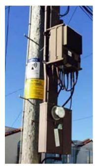
**Above:** Excess loose cabling, decals/ stickers, and cluttered appearance of equipment cabinets are not allowed.
