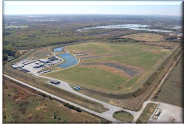
Site of future Peak Flow Diversion Structure
