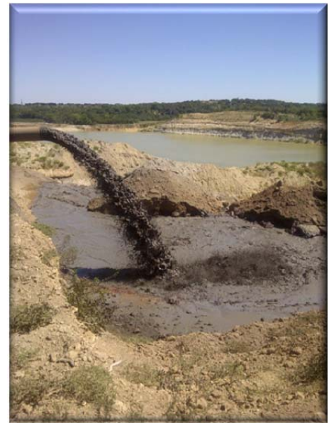
Lake Worth Dredging project
