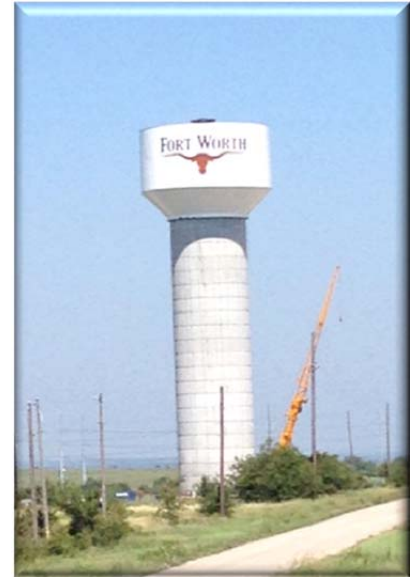
Northside IV Elevated Storage Tank
