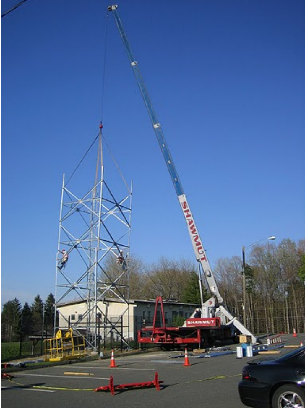
Figure 18 - A square tower is craned into place
