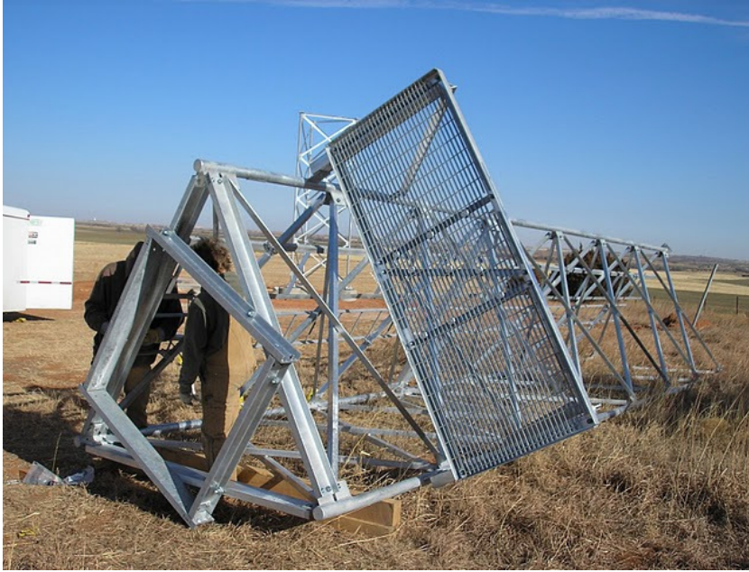
Figure 15 - Tower top with small platform
