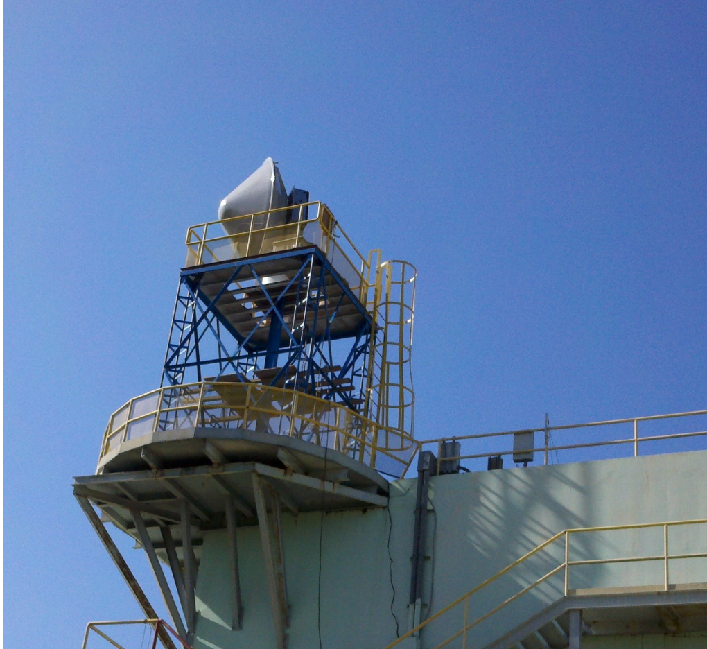
Figure 25 – Radar mounted on roof platform to clear surrounding structures. Rest of radar computing and networking equipment is housed inside the building.
