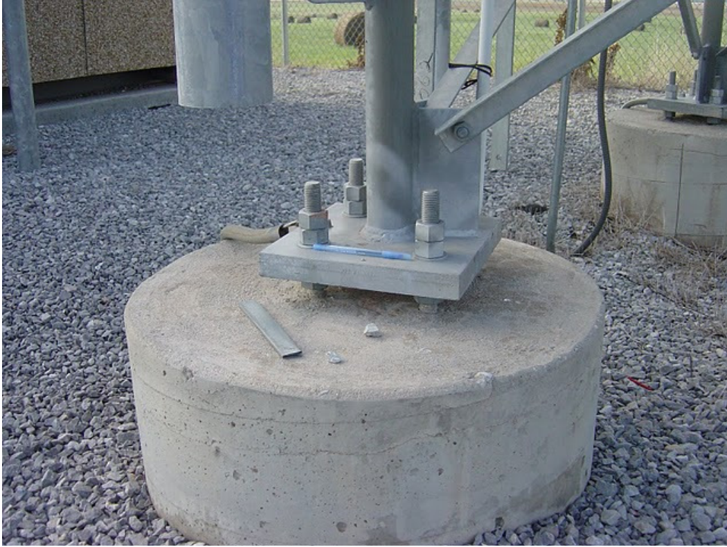
Figure 13 - Tower feet anchored to reinforced concrete cylinders.
