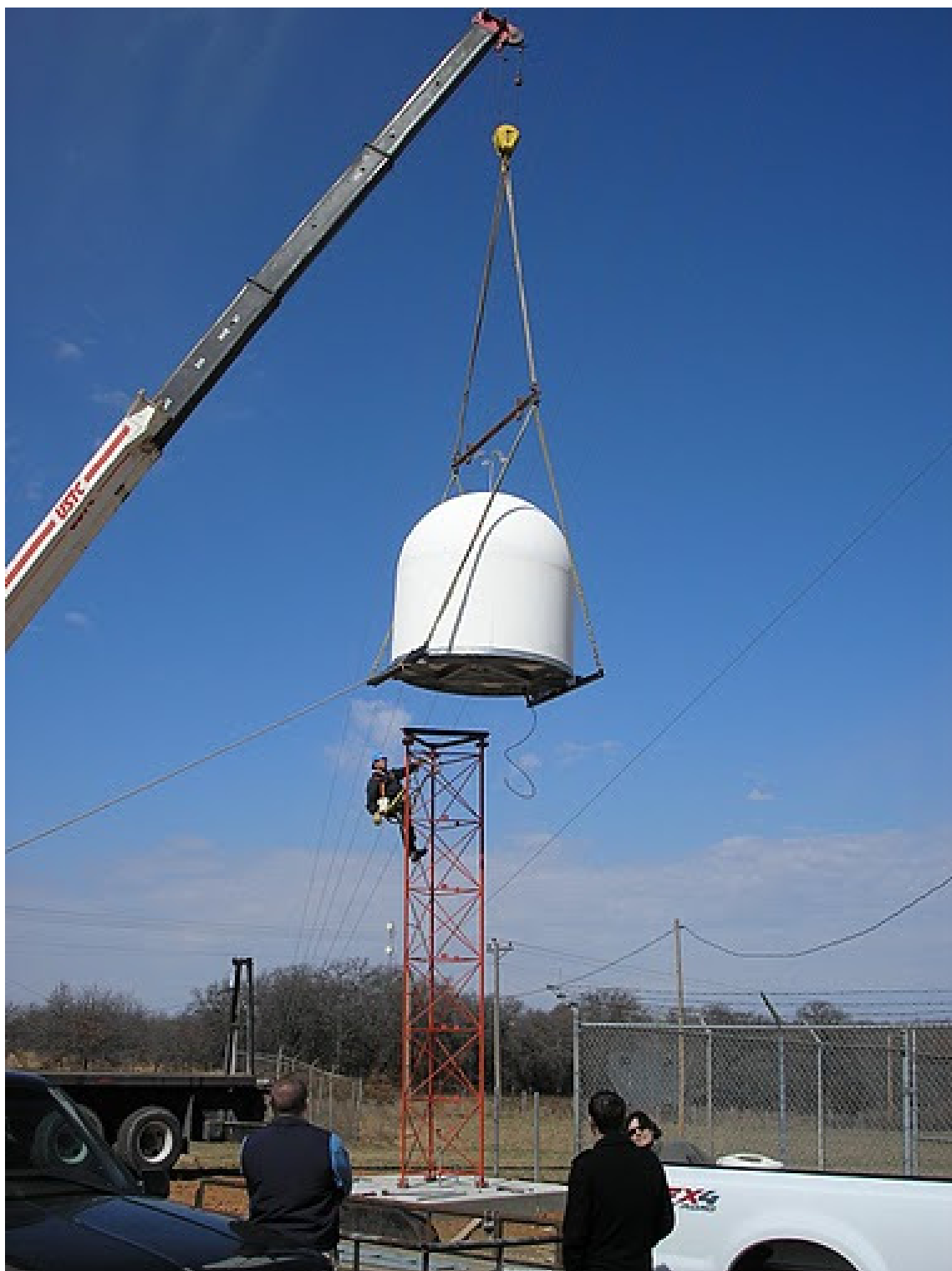
Figure 7 - Radar lifted to tower top and bolted in
