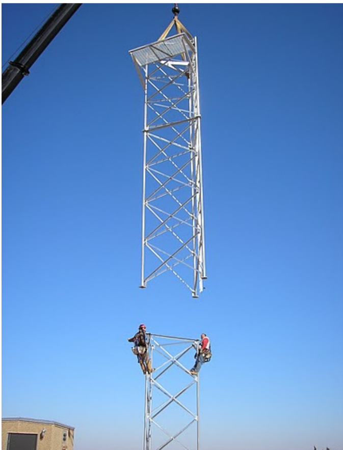
Figure 16 - Tower top craned into place
