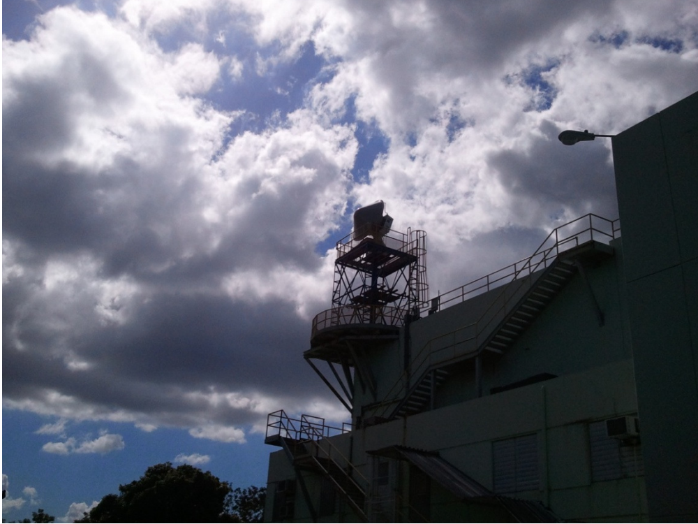
Figure 32 - Complete building rooftop installation with indoor housing for computer equipment
