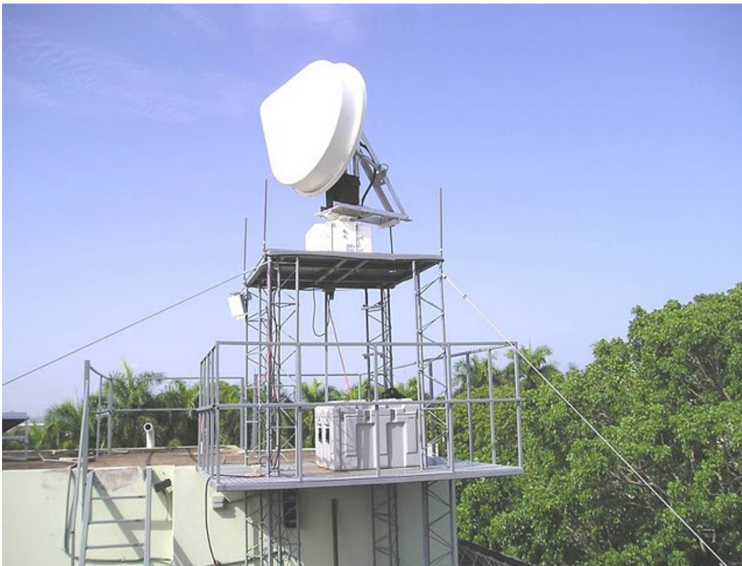
Figure 24 - Radar mounted on a small platform, elevated off a rooftop. Weatherized computer equipment housing box seen below
