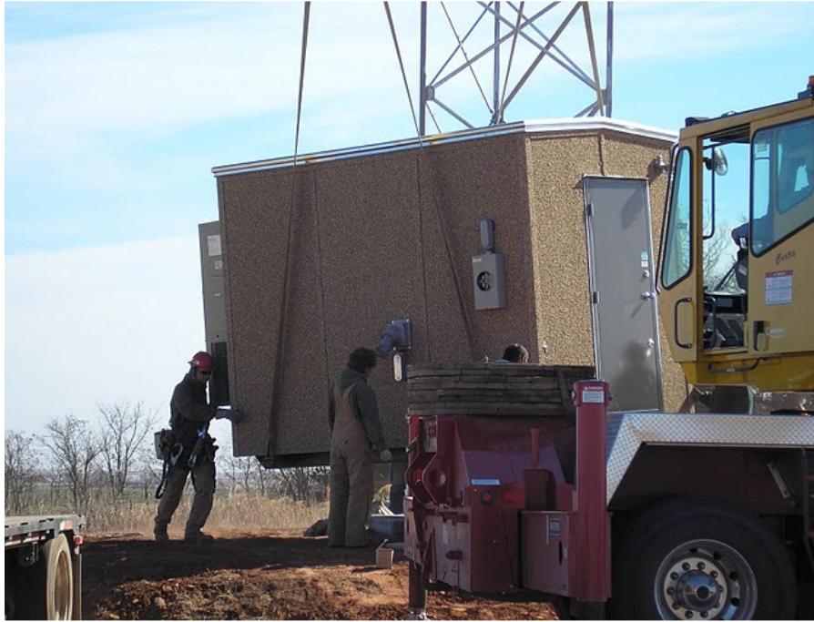
Figure 26 - A prefabricated shed is craned onto concrete slab
