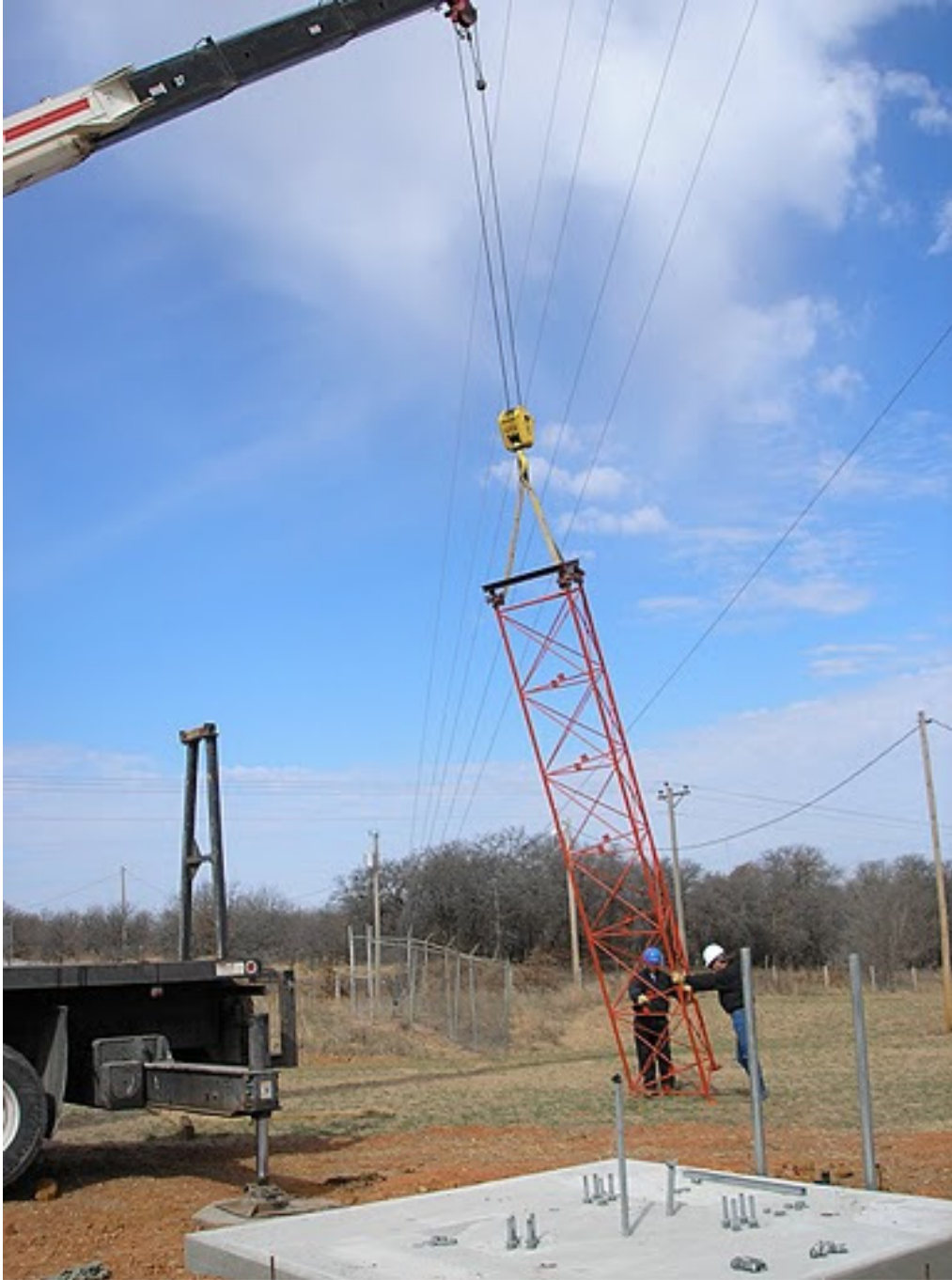
Figure 4 - Tower lifted into place
