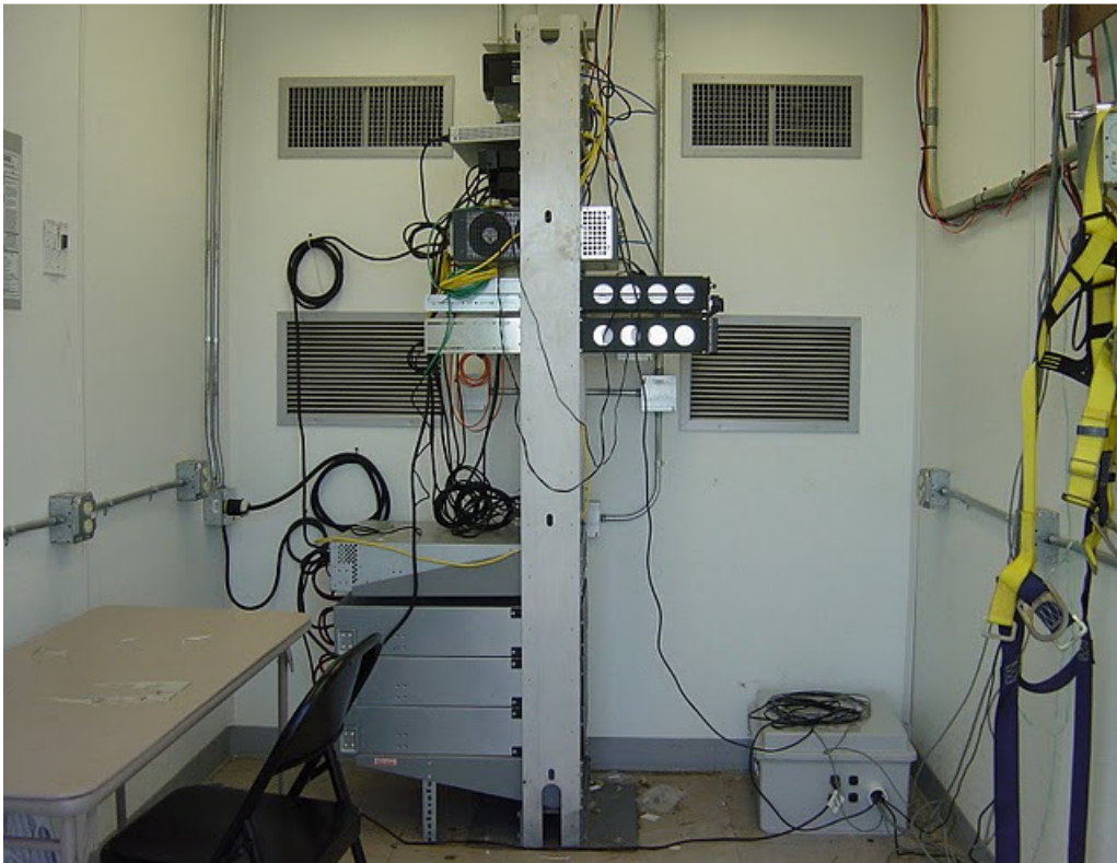
Figure 29 - Computer equipment housing installation
