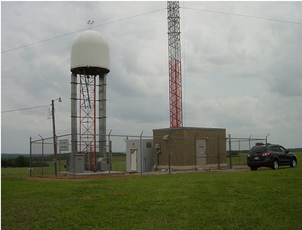
Figure 31 - Complete short tower installation with collocated existing structure for computer equipment
