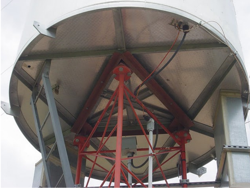
Figure 8 - Angled ladder attached to radar and tower for trapdoor entry
