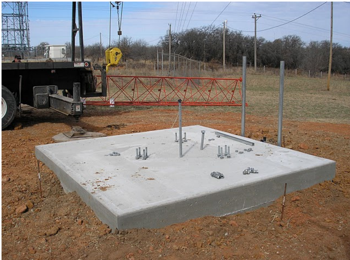
Figure 3 - Poured foundation, anchor bolts, trenched-in conduit
