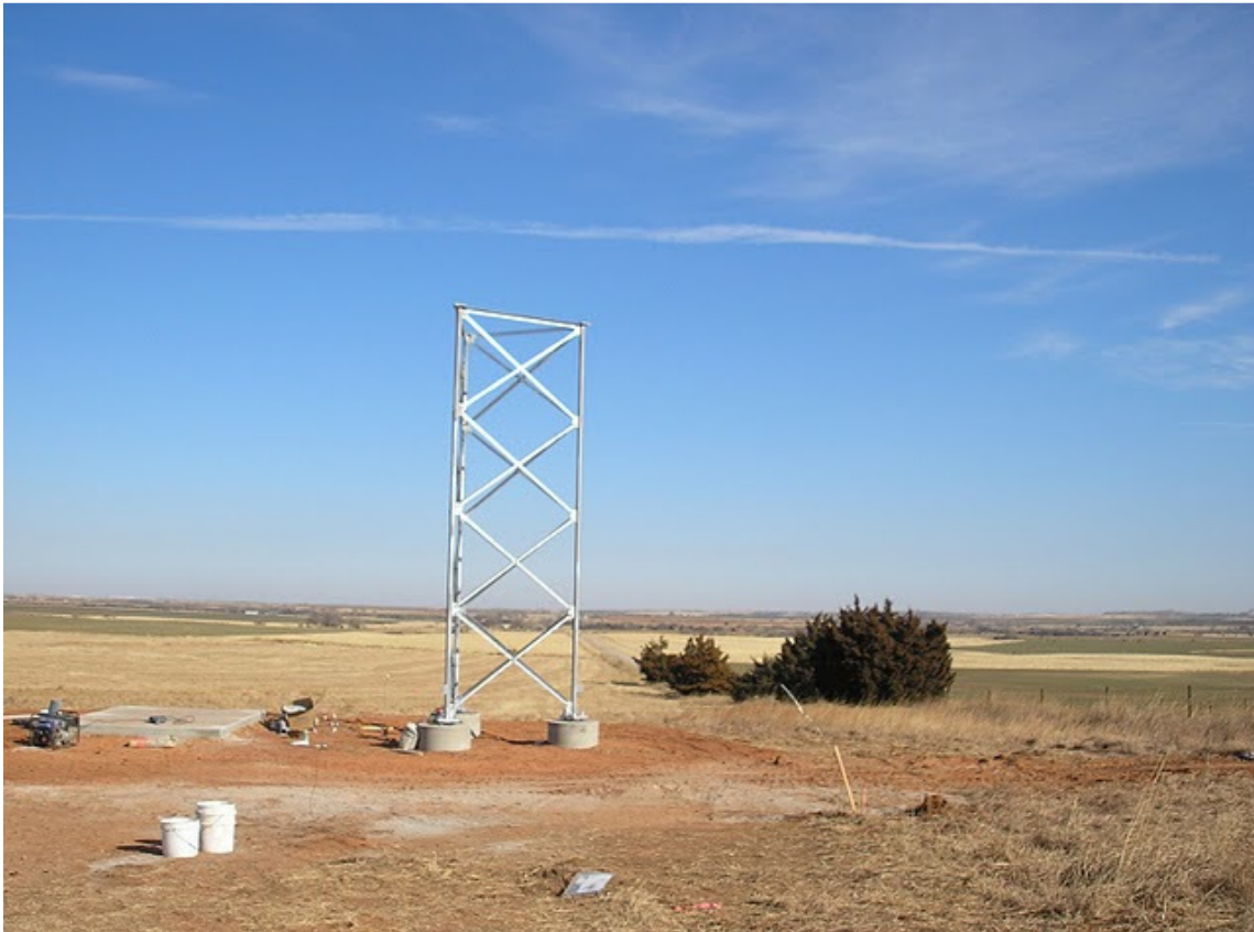
Figure 12 - Ground preparation for Tall Tower Installation
