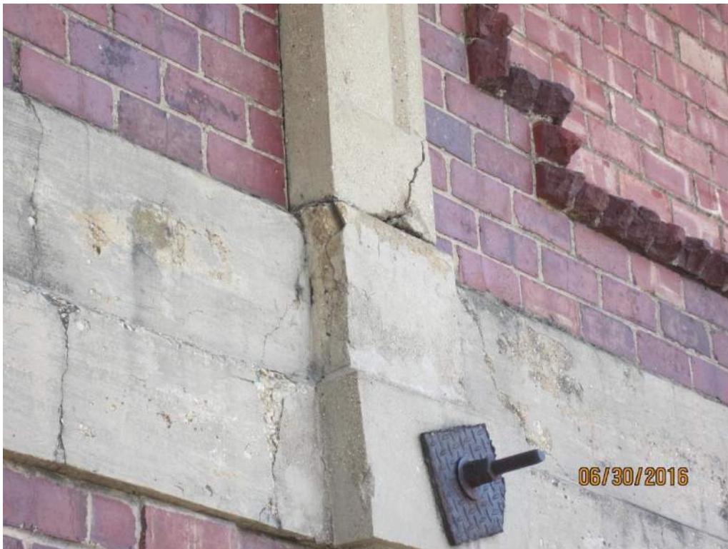
Photograph 22 – Tie-back anchor; note reveal in face of column at upper wall
