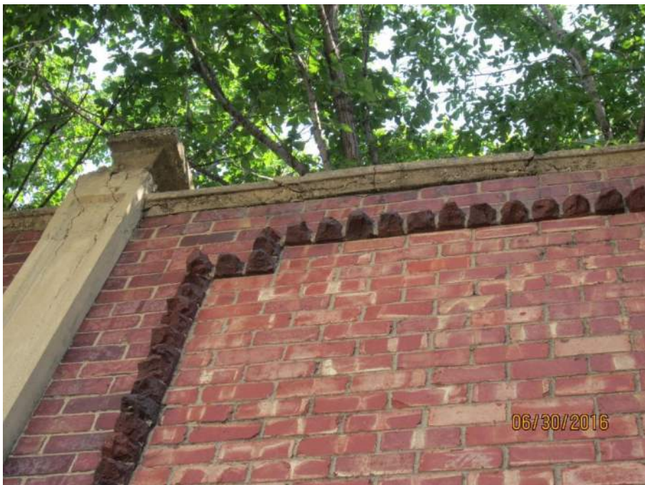
Photograph 6 – Reinforced concrete cap on top of single wythe upper masonry wall
