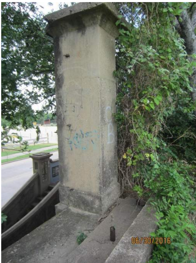
Photograph 28 – Larger columns on upper wall east of grand stairway
