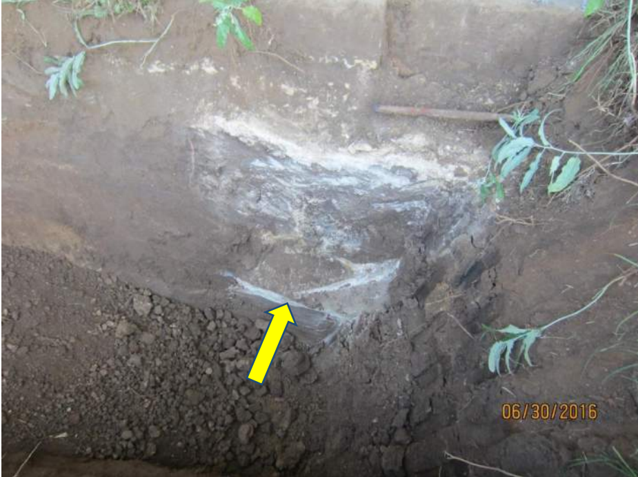
Photograph 14 – Bottom of concrete foundation on street side of wall
