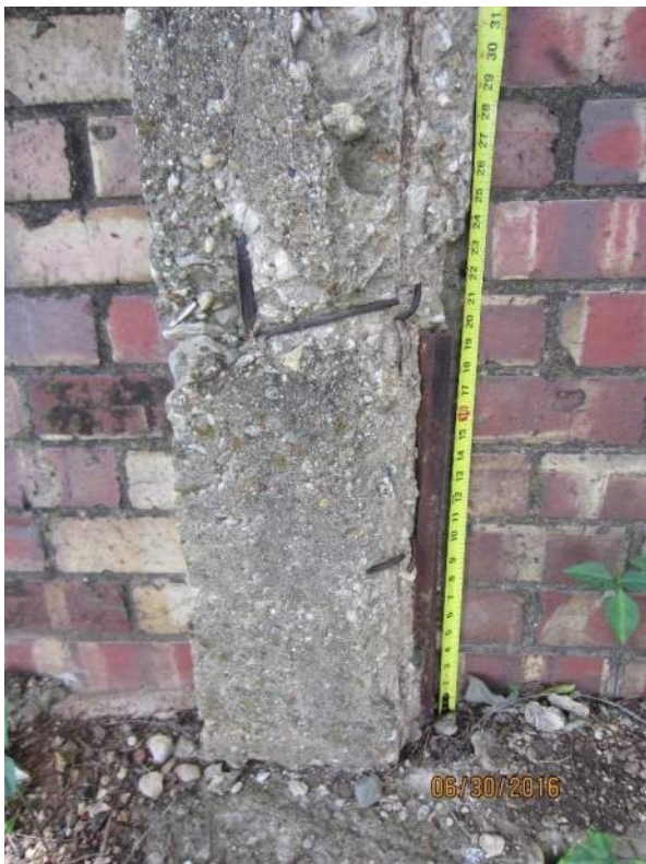
Photograph 26 – Reinforcing steel extending into upper column from pilaster below
