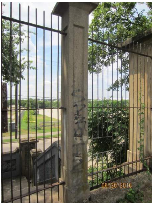
Photograph 24 – 1-inch deep reveal cast into each face of upper columns
