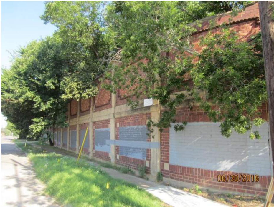
Photograph 1 – Swift masonry wall, looking west
