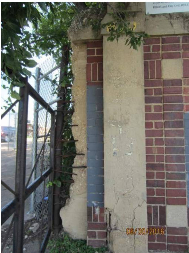
Photograph 2 – Brick veneer on reinforced concrete backup wall
