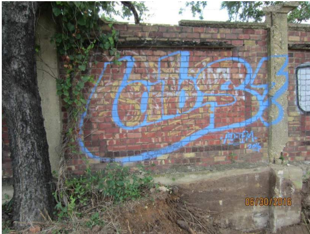
Photograph 7 – Concrete pilasters on backside of wall align with pilasters on front side
