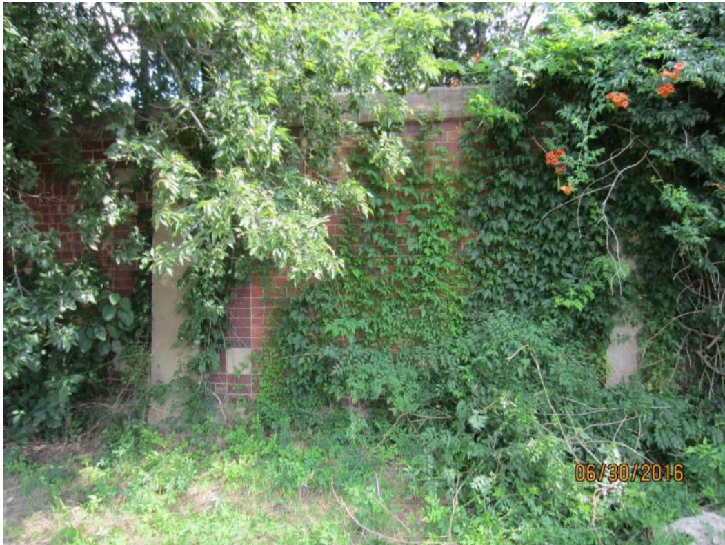
Photograph 42 – Vegetation along south side of wall
